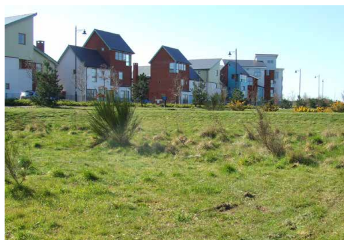
SuDS dry attenuation area
